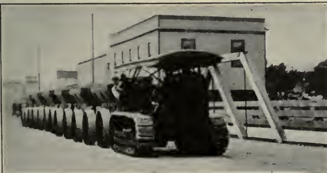
HAULING GRAVEL TO HIGHWAY JOB
